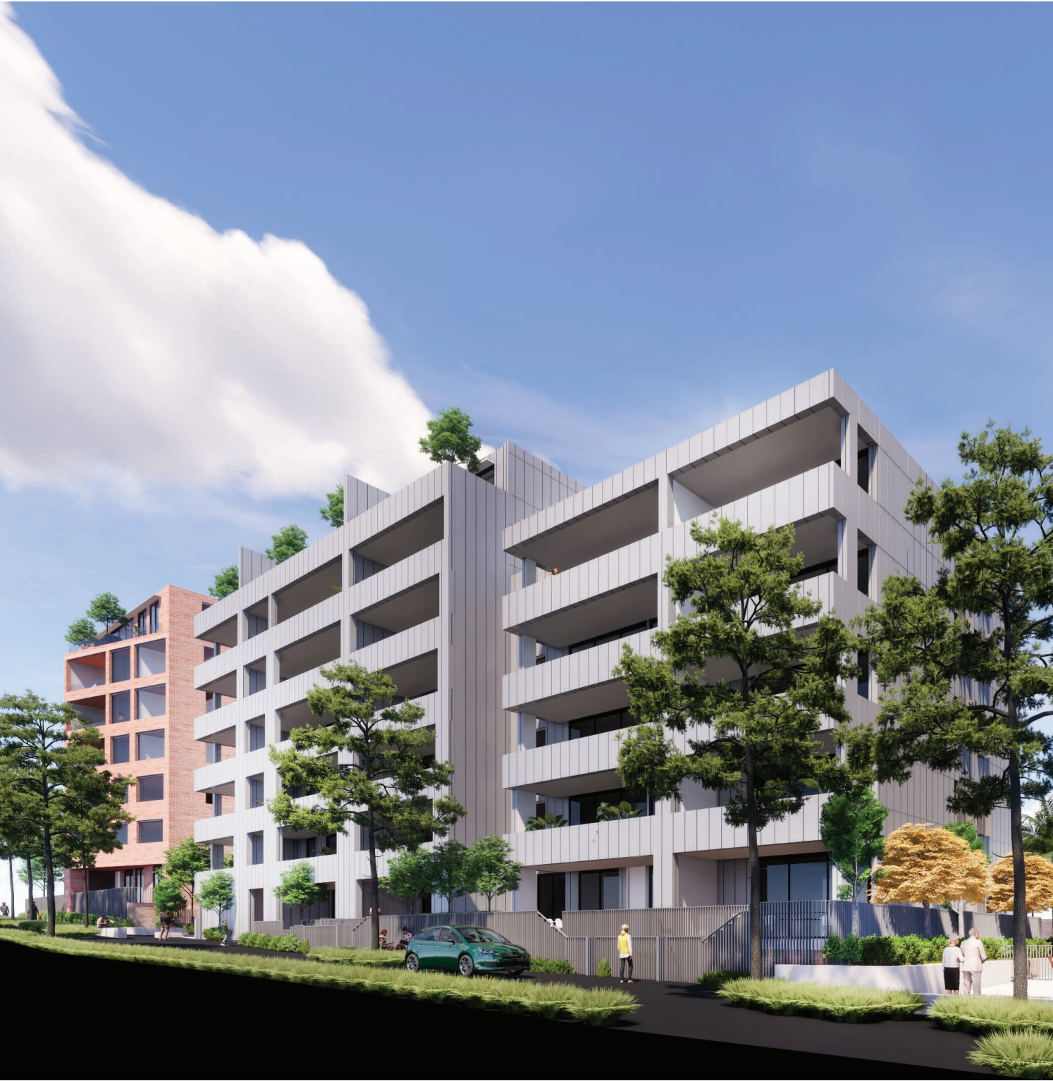
Silver Grey Profiled Metal Cladding
